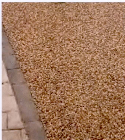
Stabilized aggregate reduces storm runoff from low-traffic paving areas.
