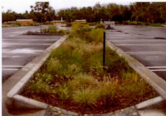
Vegetated swales accept stormwater for conveyance, storage and infiltration.
