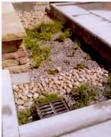
Bioretention cells fit into constrained urban site.
