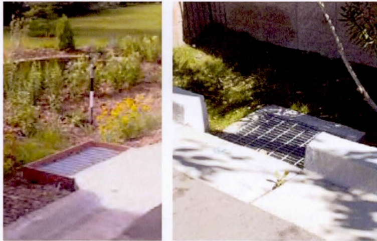
Sediment capture can be open or covered.
