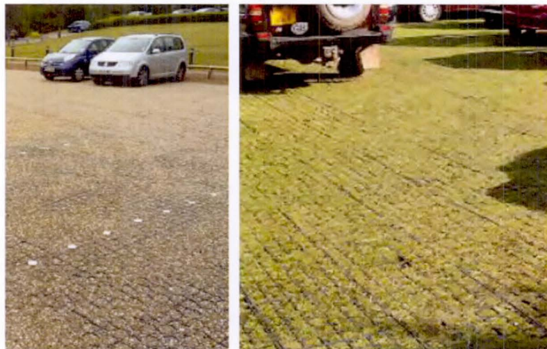
Structural grid paving reduces runoff in parking areas and firelanes.
