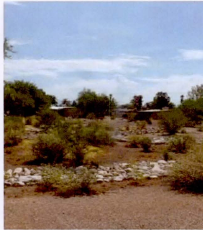
Bioretention areas detain stormwater while enhancing the landscape.
