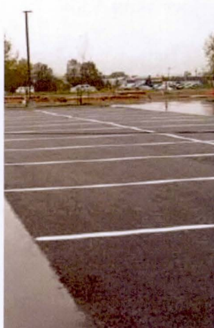
Porous asphalt paving is a runoff-reducing in paving areas and driveways.
