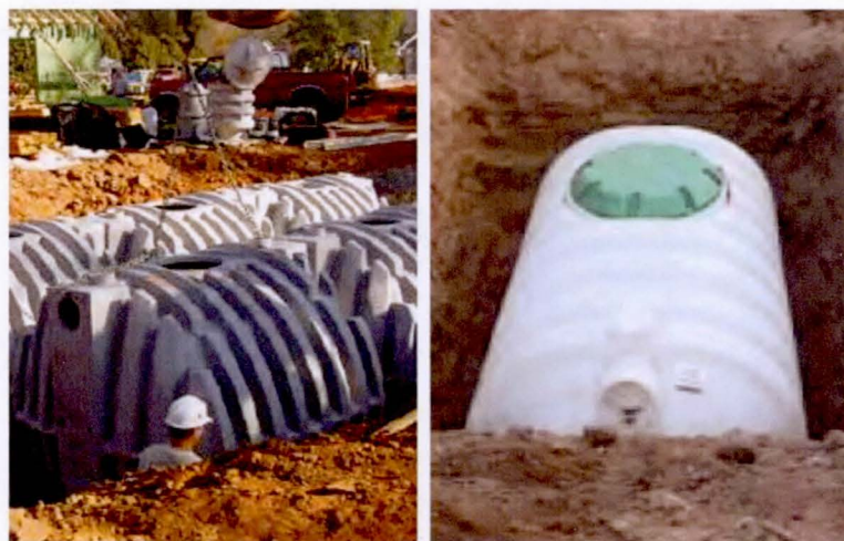
Underground cisterns provide storage areas for rainwater reuse.
