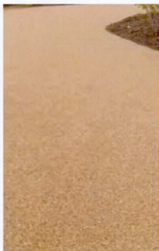
Stabilized aggregate reduces storm runoff from low-traffic paving areas.
