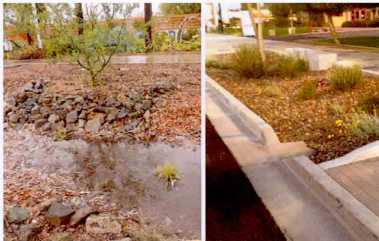
Vegetated swales accept stormwater for conveyance, storage and infiltration.
