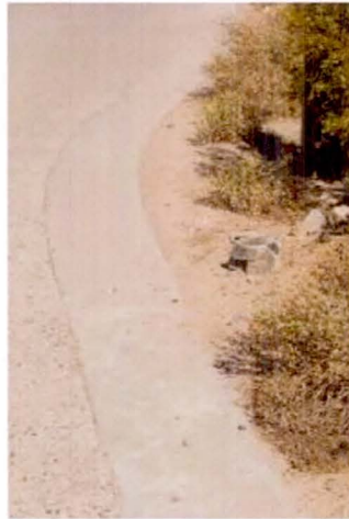
Flush curbs allow stormwater to sheet drain to landscape areas.
