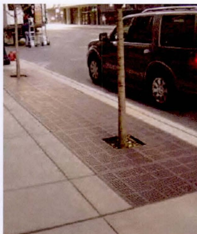
Bioretention planters provide stormwater storage and promote healthy growth of trees and plants.
