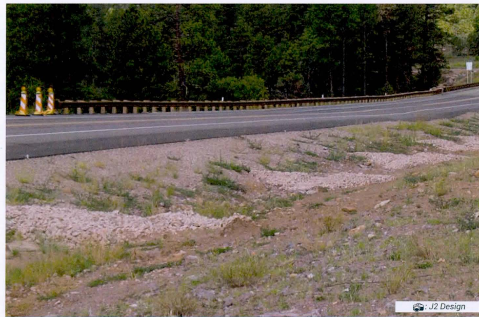
Example of Rainwater Check Dams
