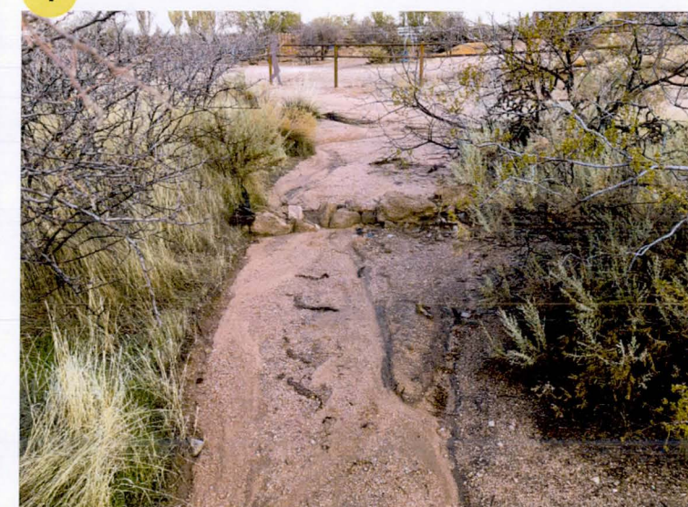
Make Shift Check Dam Constructed with Rip Rap
