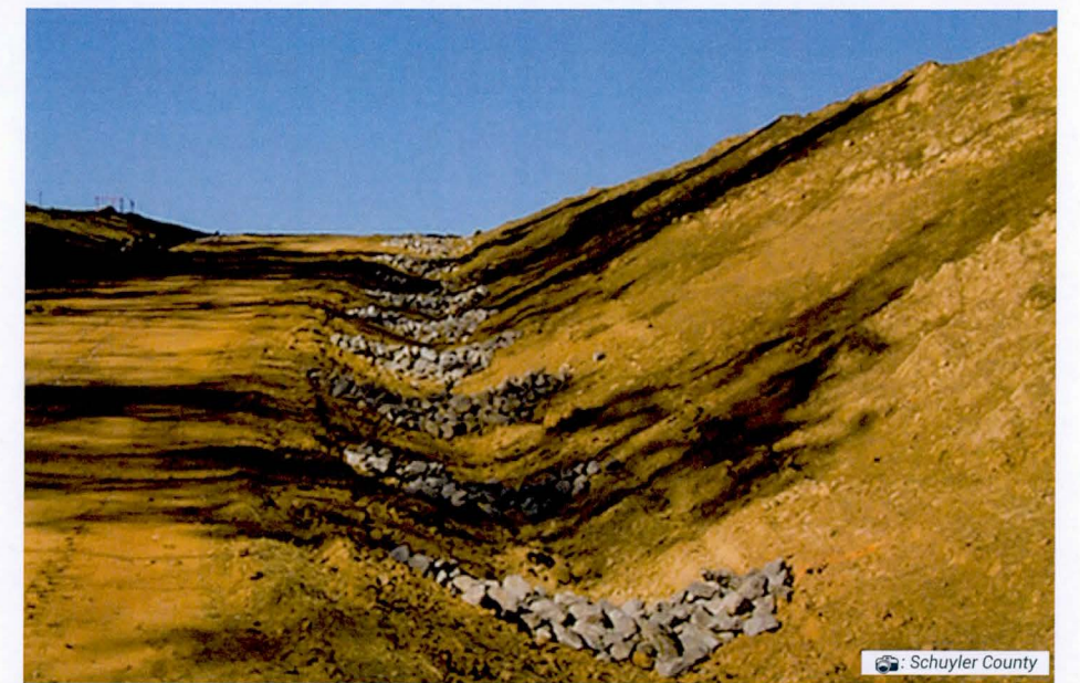
Example of Rainwater Check Dams
