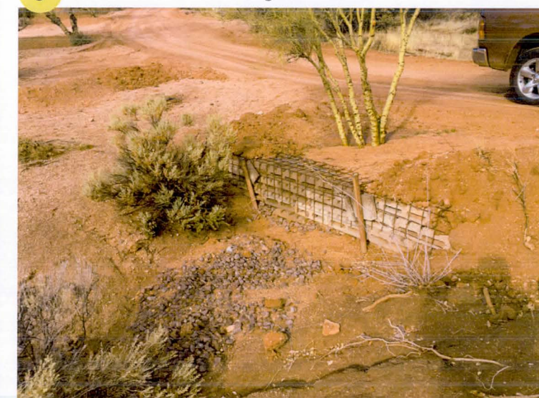
Make Shift Check Dam Constructed with CMU Block
