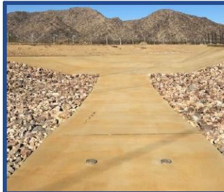
Concrete stain that will blend to a natural earth tone overtime.
