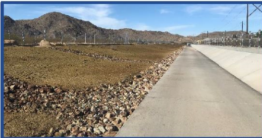
View of channel and improvements looking northbound
