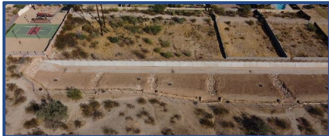
Aerial view of the completed construction site
