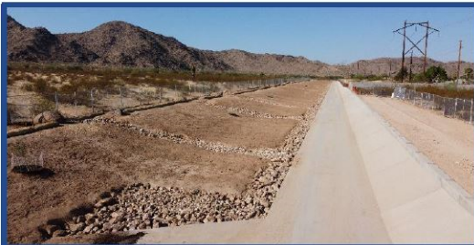
View of channel and improvements looking northbound
